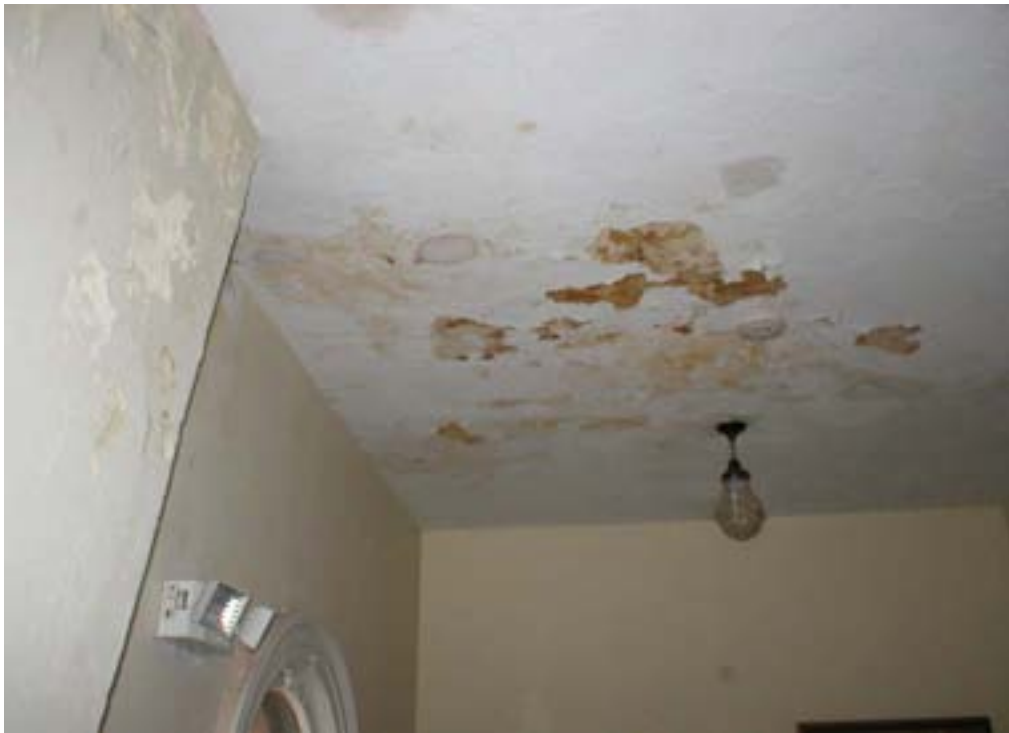
#3 Water damage below these roof areas.
