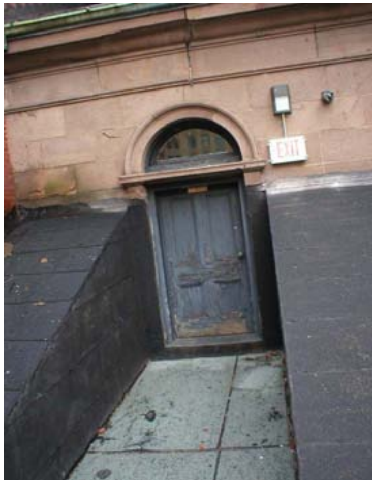
#2 Parish Hall roof areas and door. Both need replacement.
