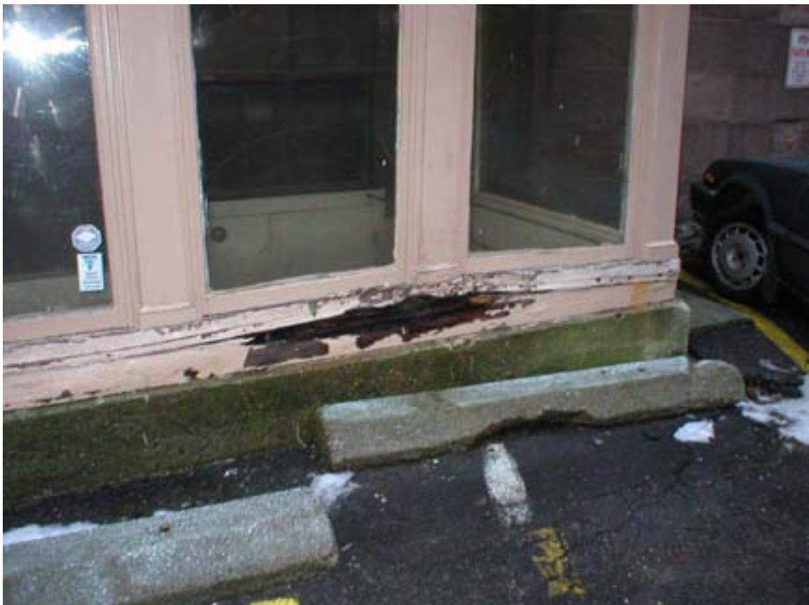
#6 Right side entry to basement level damaged and decayed. Needs rebuilding.
