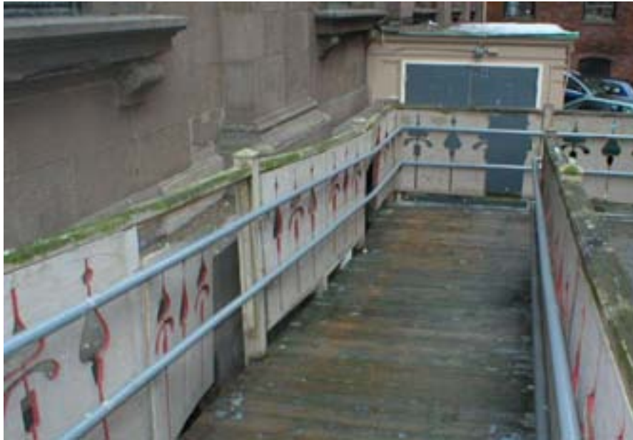
#5 Right side ramp and railing deteriorated and needing rebuilding.
