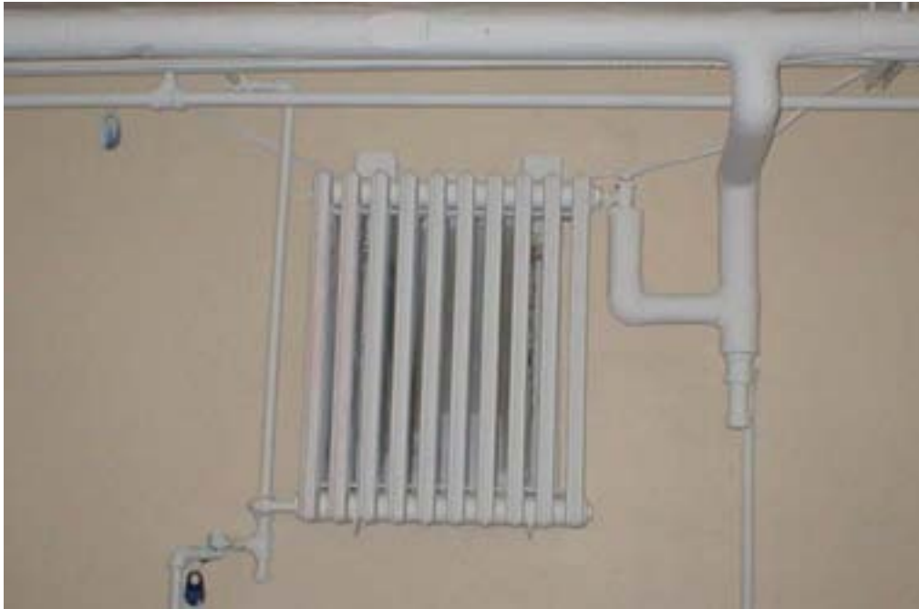
#7 Steam radiator for heat distribution in basement.
