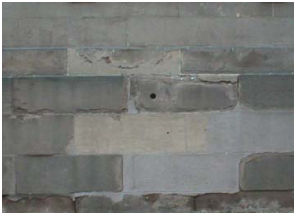
#4 Exterior masonry deterioration.
