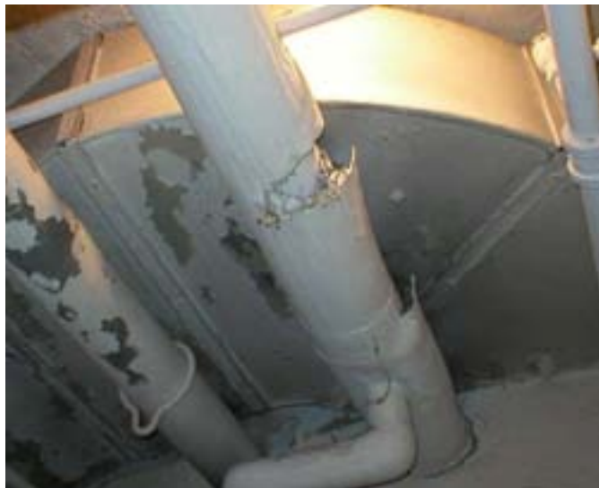
#8 Possible asbestos containing material with damage. Evaluate and abate as needed.
