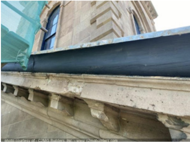
Wood stripping at pediment cornice — old growth timbers still intact!
