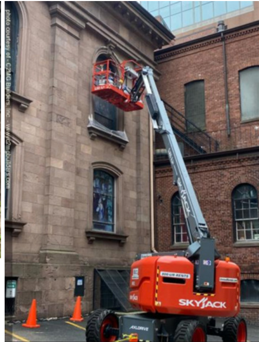
Stripping/painting/glazing of upper Tiffanys
